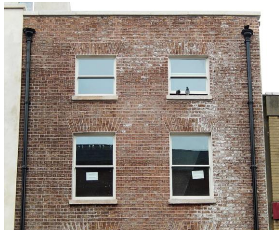
View of new sash windows and repointed facade
