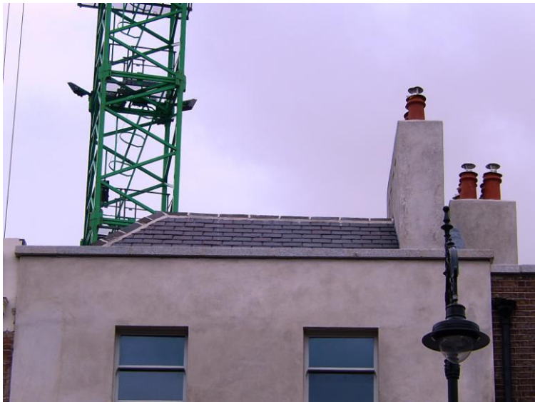
View of front roof elevation surviving steeply pitched roof with large chimneystack
