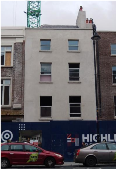
View of front elevation in 2012 prior to present works
