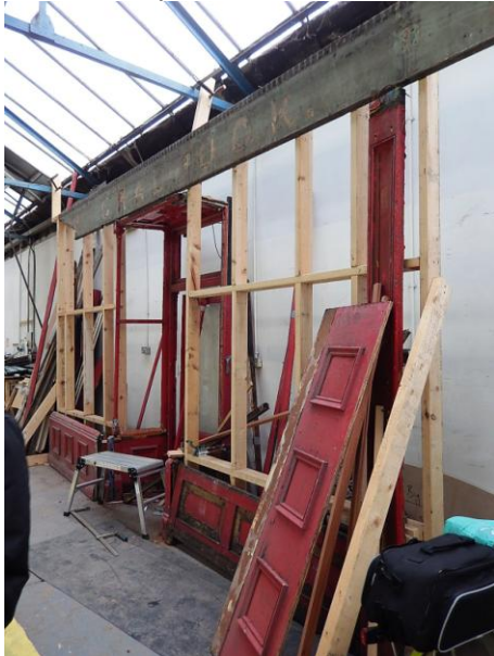
View of shopfront (originally from number 32 prior to repair in joiners workshop and shortly after installation in number 33)
