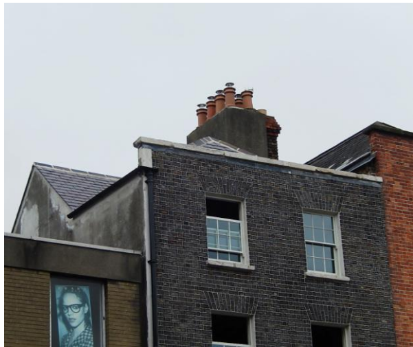
View of the cruciform roof and substantial chimney stack
