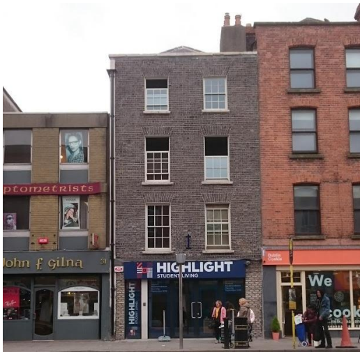
View of front elevation with recently repointed facade with wiggled detail
