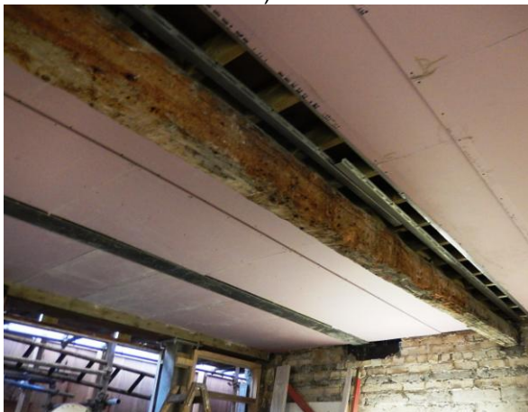
View of bressumer beam to ground floor
