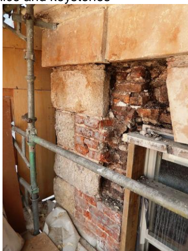
Portland cornice and granite quoin stone detail
