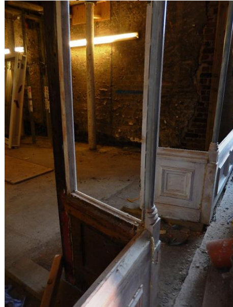
View of shopfront (originally from number 32 prior to repair in joiners workshop and shortly after installation in number 33)
