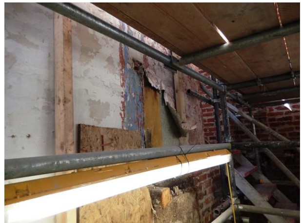
View of internal stairs hall wall to be repaired
