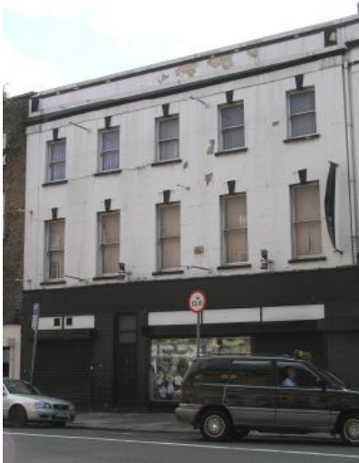
View of front facade prior to recent works
