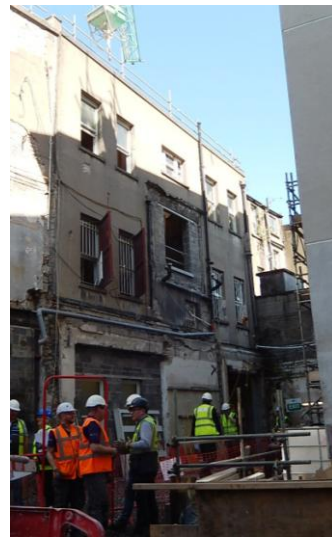
Rear elevation with largely rebuilt facade
